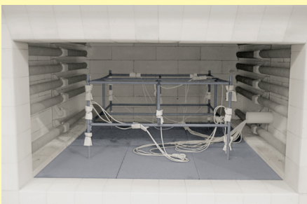
Measurement set-up in an annealing furnace
