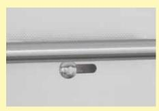
Adjustable air inlet integrated in the door
