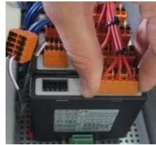
Fig. 11: Installing the controller module (similar to picture)
