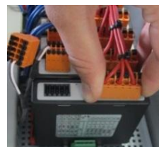
Fig. 13: Installing the controller module (similar to picture)
